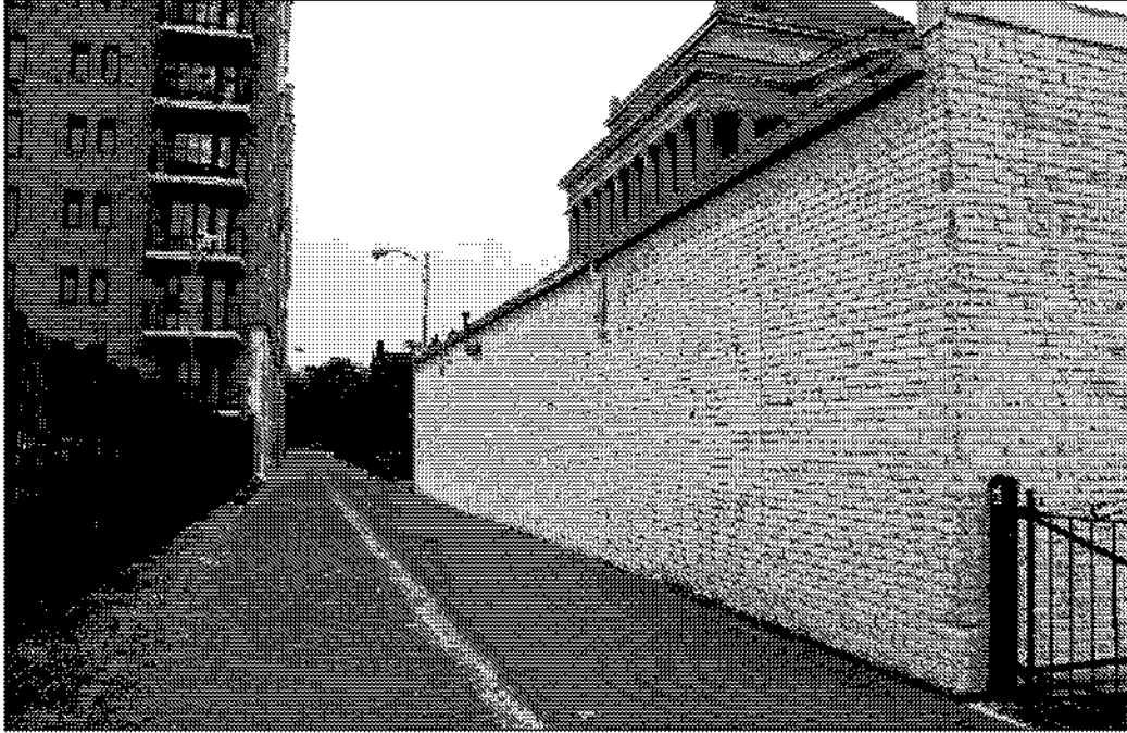
Figure 3: Scottish Rite Temple Garage, south elevation, facing northwest. EHT Traceries.
