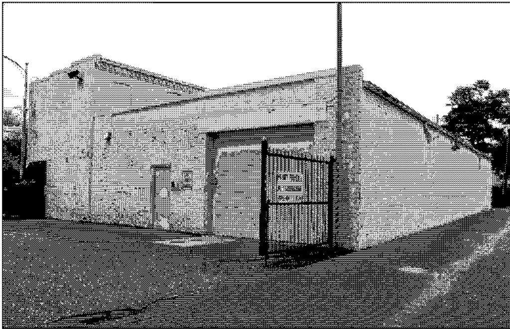
Figure 2: Scottish Rite Temple Garage, west and south elevations, facing northeast. EHT Tracerics.
